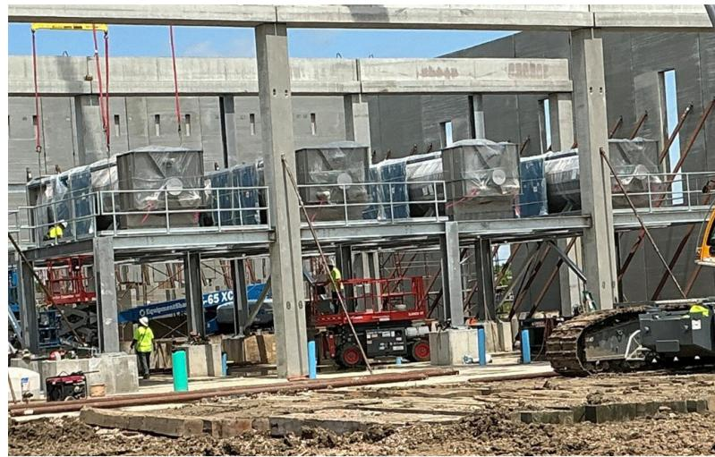
**June 2025:** Four screw presses were installed into the Dewatering Building. Screw presses separate solids from the liquid that comes from the Solids Holding Tank for disposal. The remaining liquids are recycled back into the treatment process.
