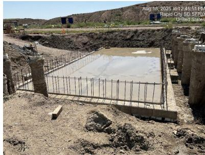
The concrete slab for the lower level of the South Electrical Building is placed.
